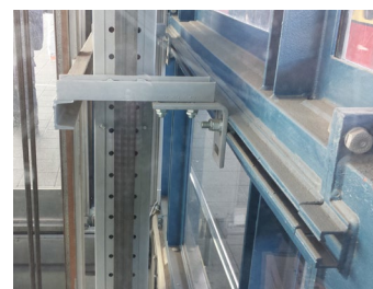
PEC framing channels can be welded directly to the steel components
