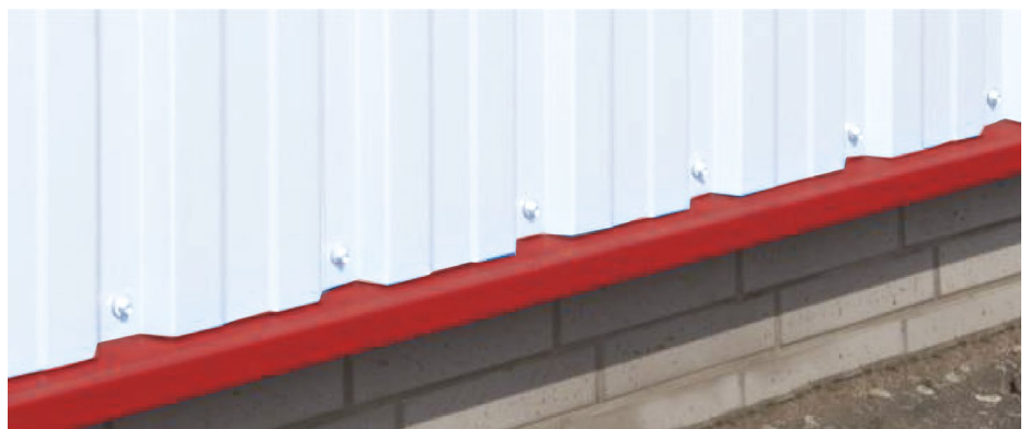
Examples for the attachment of trapezoidal sheets with PEC-TU
